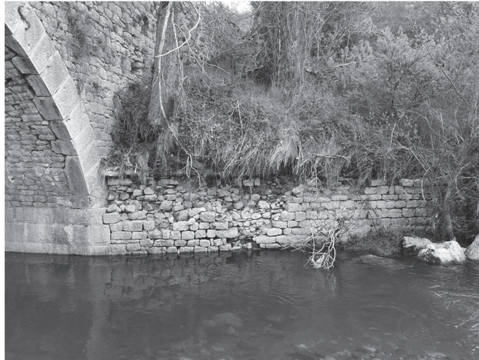
Fig. 7: Shen Prodhomi Brige, retaining wall (IMK)
